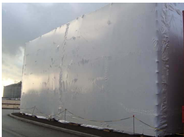
ECHAFAUDAGE - CONFINEMENT THERMO-RETRACTABLE
